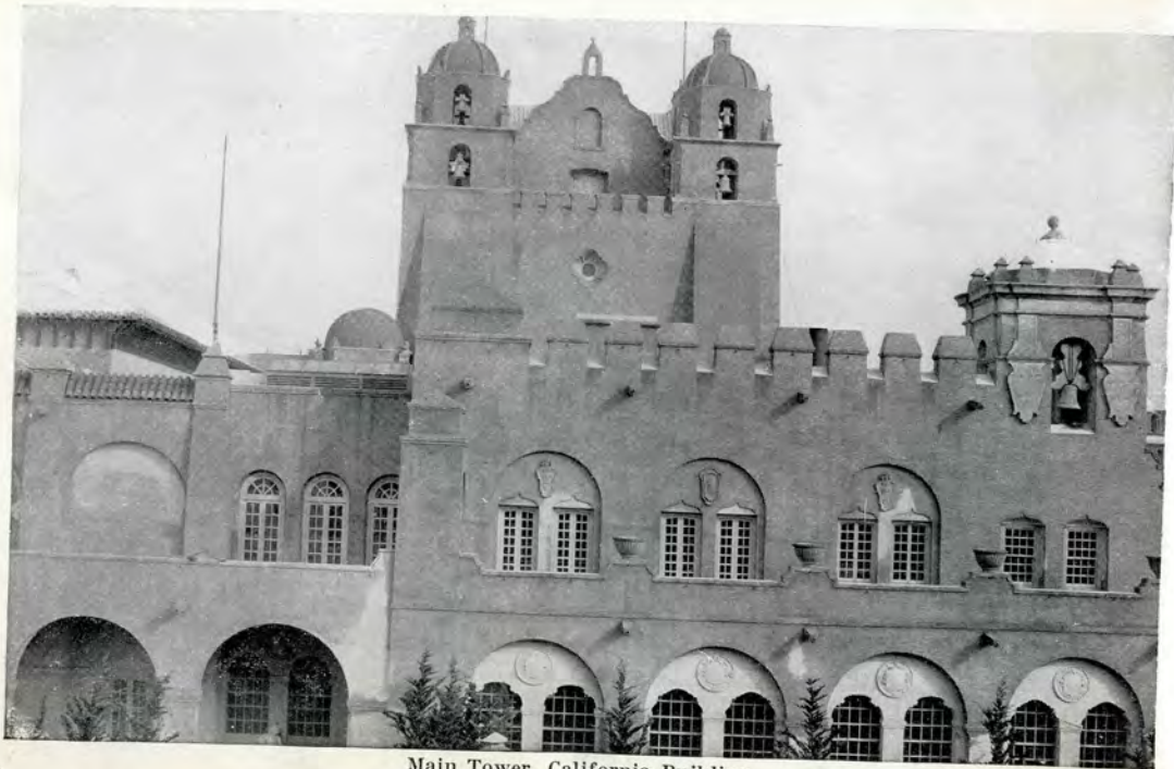
Main Tower, California Building
