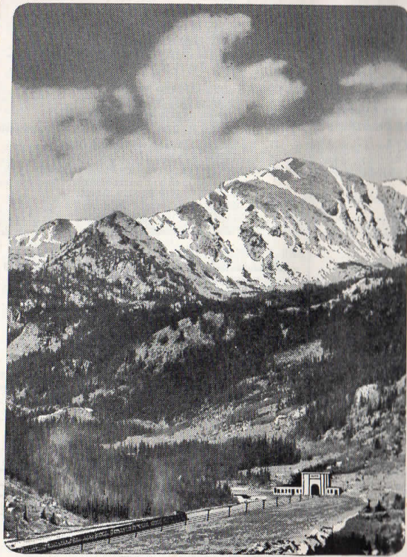
East Portal, Moffat Tunnel
