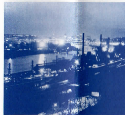
Lighting Up the Night Sky— Steel Mills in Pittsburgh
