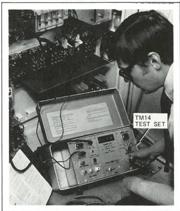
FIG. III-50. CHECKING FL182 PANEL USING TM14 TEST SET.
