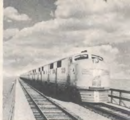
CROSSING GREAT SALT LAKE on the historic Overland Route
