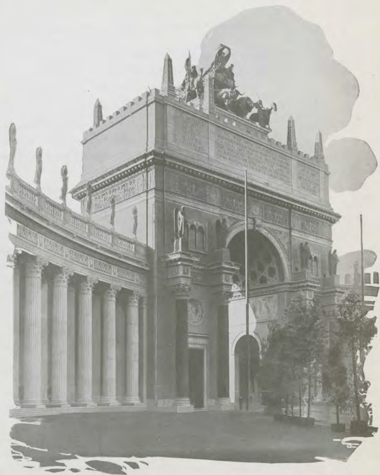
Arch of the Setting Sun, at the west entrance of the Court of the Universe.
