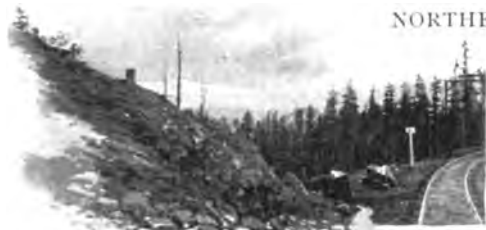
APPROACHING TUNNEL NO. 2, CASCADE MTS.
