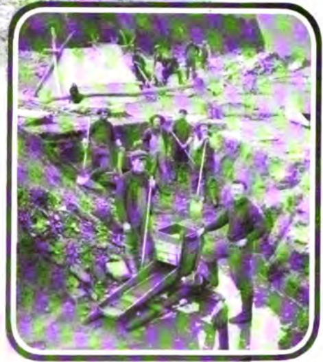
A gold rocker. Second stage of placer mining.
