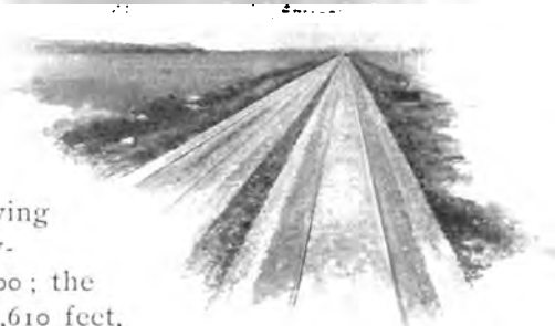
Northern Pacific Stone Ballasted Track
