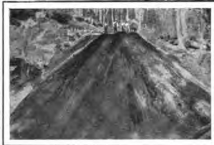
Track Grading. End of a Dump.
