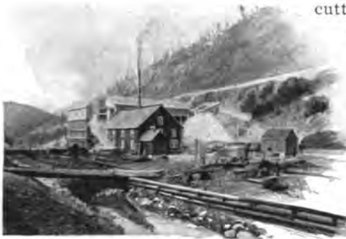
AIR COMPRESSOR, STANDARD MINE, BETWEEN BURKE AND GEM, IDAHO.
