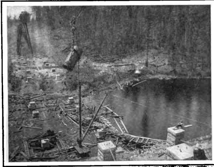
Constructing "Granite Trestle" (Steel), Idaho. Showing Piers.
