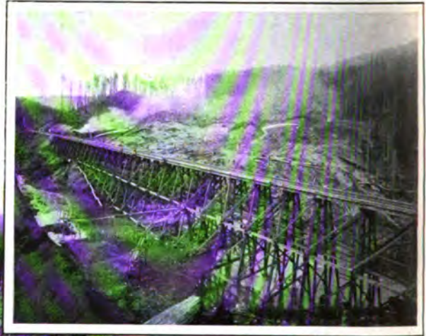
Sluicing Down the Mountains and filling Trestle by Means of Giant Nozzles.
