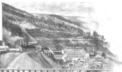
DRUM LUMMON MINE AND MILL, MARYSVILLE, MONT.
